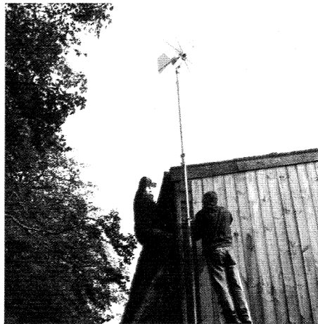
Keith, G7NBU & Allan, G1JXI rig the turbine.
